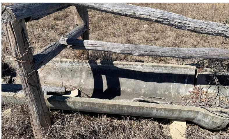
Figure 47. Detail of the trough's timber post-and-rail frame. Note the concrete footings.
