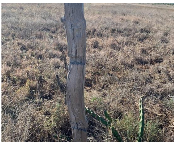
Figure 83. One of the remnant timber posts located at WS26-4. Note the two rectangular notches, which indicate that sections of this former fence line may have also been constructed using timber rails.
