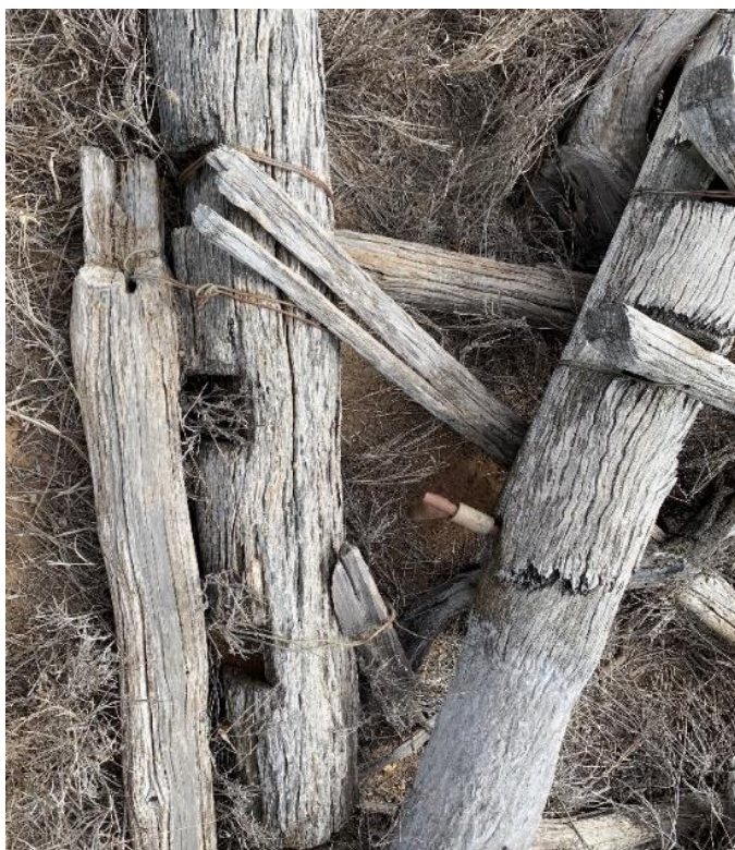
Figure 30. Detail of the timber fence posts comprising WS05, some of which have been mortised for rails.
