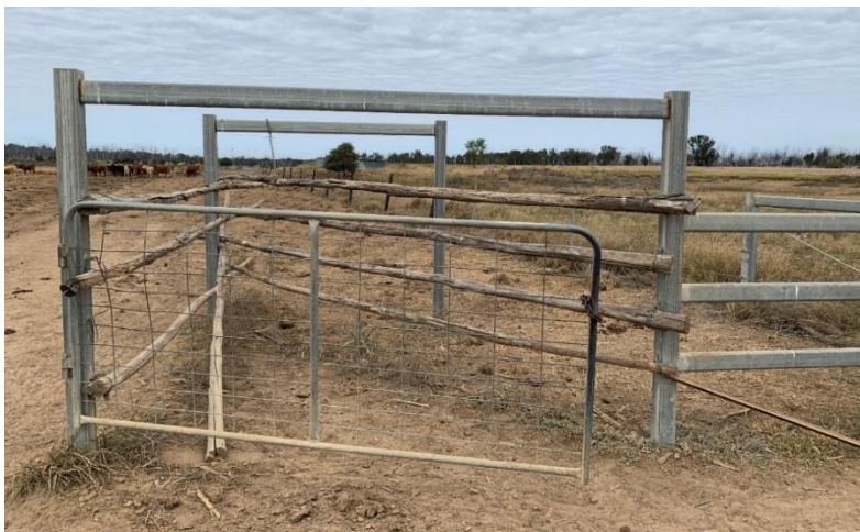
Figure 21. Detail of the main cattle sorting gate of WS02. Note that the gate's sorting component is constructed of timber rails supported within a modern metal framework.
