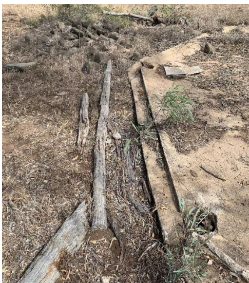
Figure 36. View of the eastern edge of the concrete slab, showing the lipped edge and the holes on each corner, which may be indicative of former posts or drainage holes.
