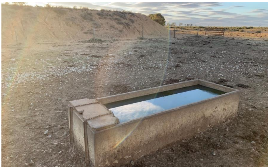
Figure 92. View north-west showing the concrete water trough adjacent to the dam at WS30. The steep dam embankment, surrounded by a timber post and wire fence, is visible behind.
