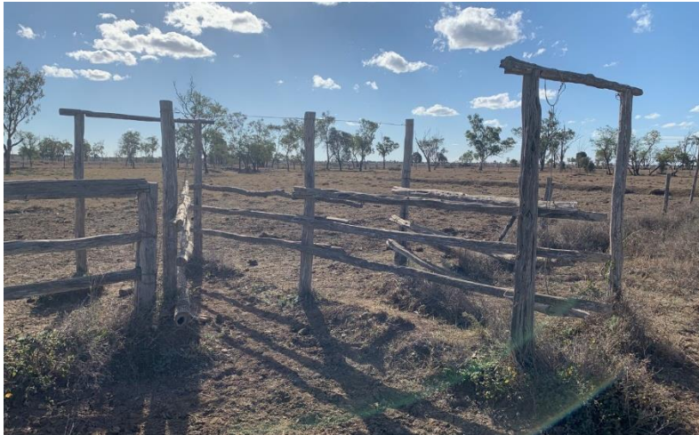
Figure 79. View north-west showing one of the cattle sorting gates at WS25. Its construction is timber post-and-rail bound together with metal wire.
