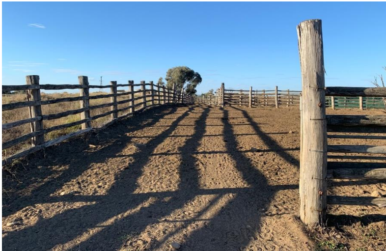
Figure 86. View north showing the interior of the main holding yard at WS27. Note the consistent use of timber post-and-rail for the construction of the fencing.
