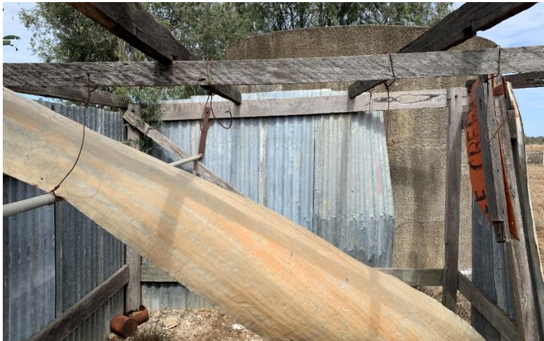
Figure 32. View south showing the interior of the pump shed, which is in a state of partial collapse. Note the large corrugated iron roof sheet, which has collapsed into the interior of the shed.
