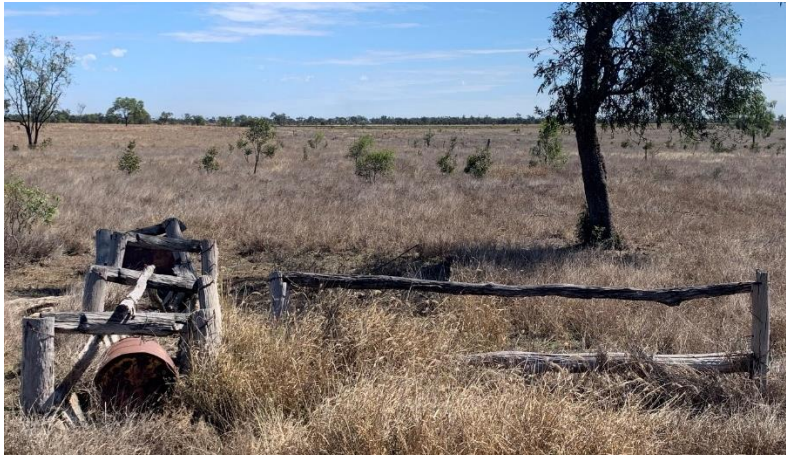
Figure 49. View west showing WS12, a concrete water trough with a timber shell and surrounded by a timber post-and-rail frame. Note the remains of a timber post-and-rail fence perpendicular to the trough.
