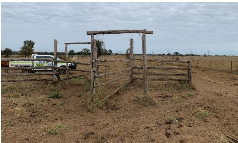
Figure 18. View west showing timber gate apparatus at WS01. Note the timber post-and-rail construction.
