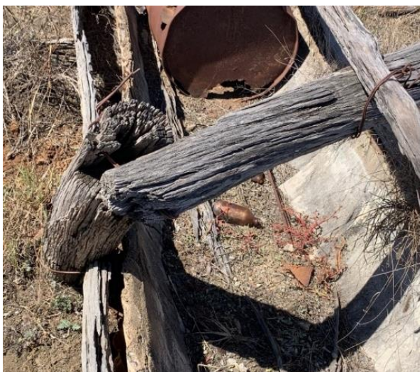
Figure 51. The eastern end of the water trough, showing the timber shell encasing the concrete trough.
