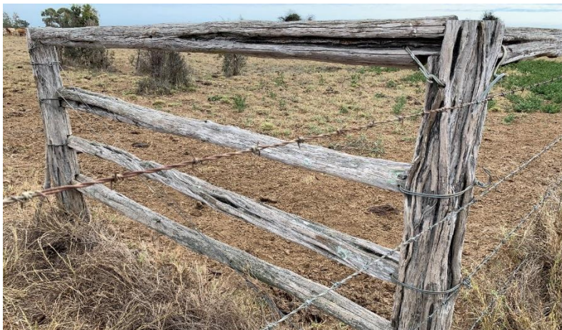
Figure 19. The timber cattle yard fencing typical of WS01, illustrating the timber post-and-rail construction.
