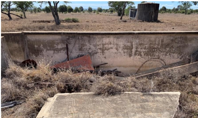
Figure 38. The collapsed southern wall (foreground) and the extant northern wall of the former cattle dip.
