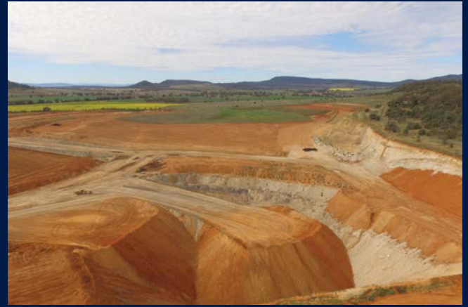
July 2020 final stages of backfilling & topsoil spreading
