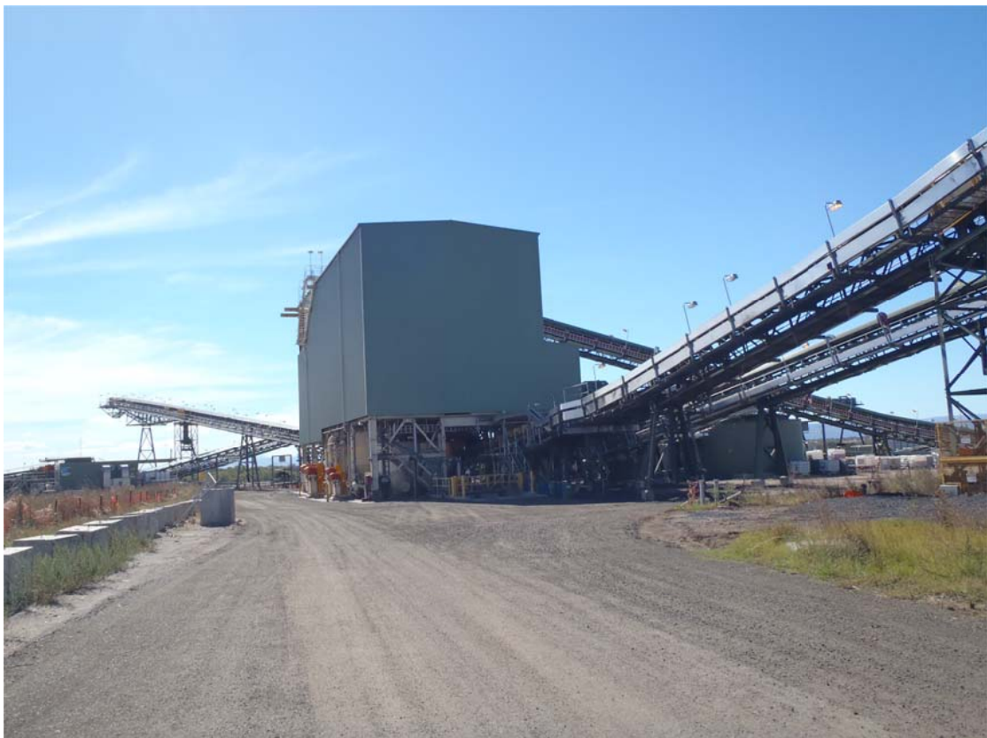
Plate 2 - Coal Handling and Preparation Plant
