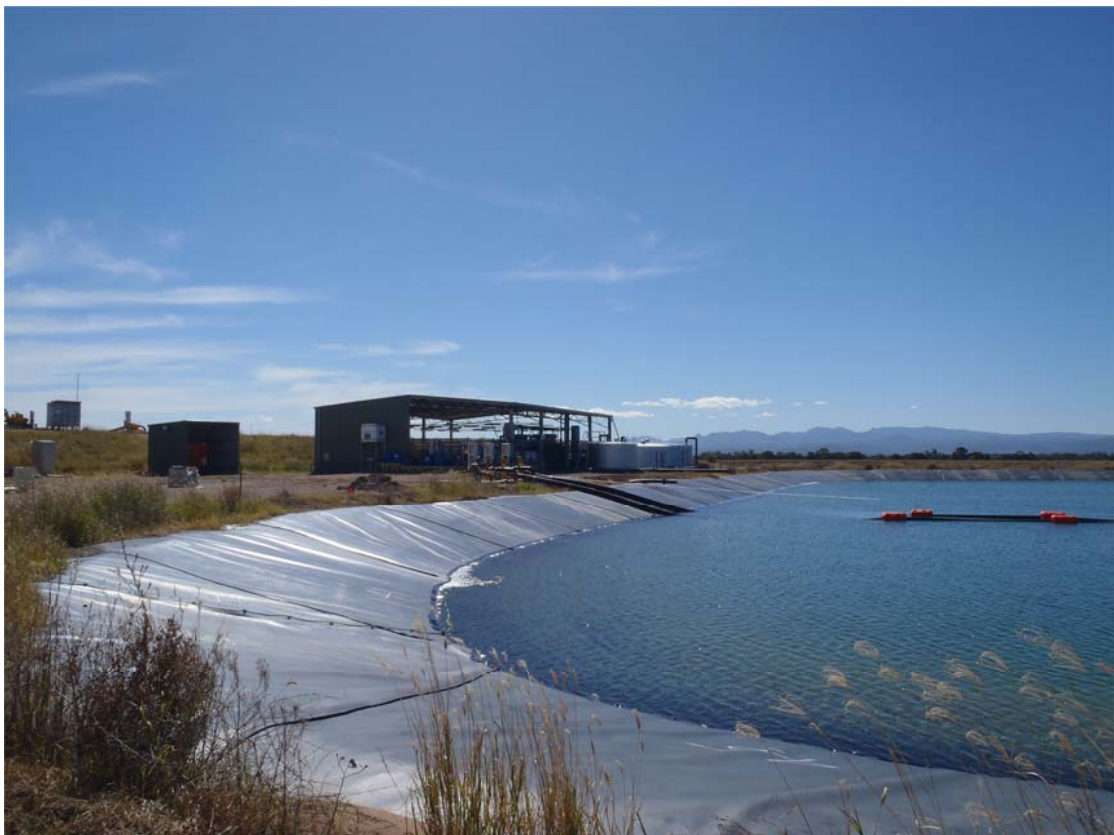
Plate 4 - Water Treatment Plant (Undergoing Commissioning)
