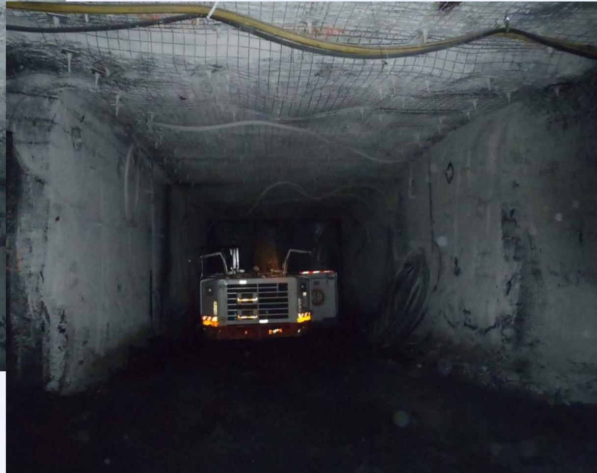
Development roadway dimensions 5.4m wide x 3.5m high
