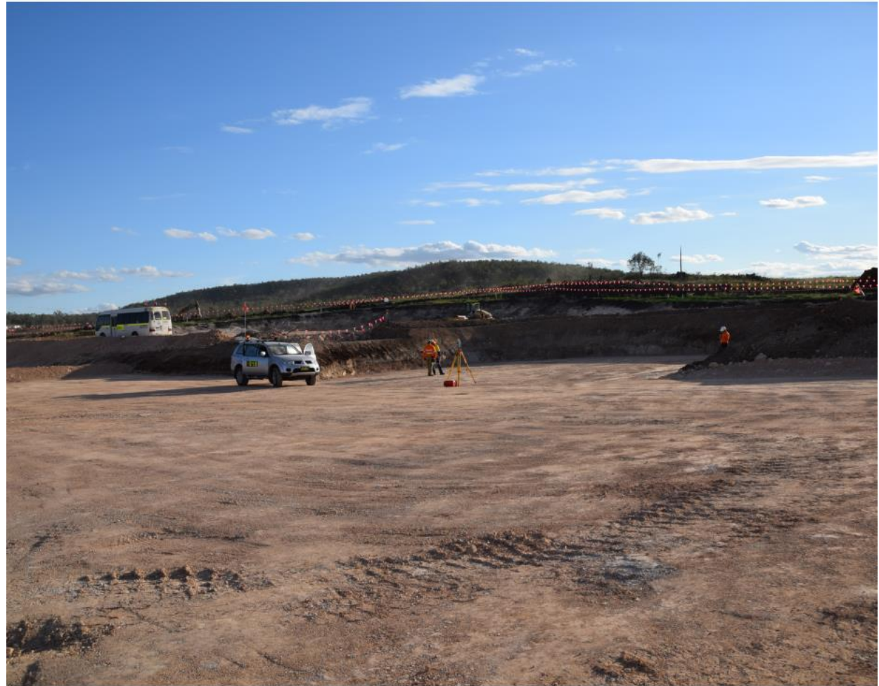
TLO Platform Complete ready for Piling
