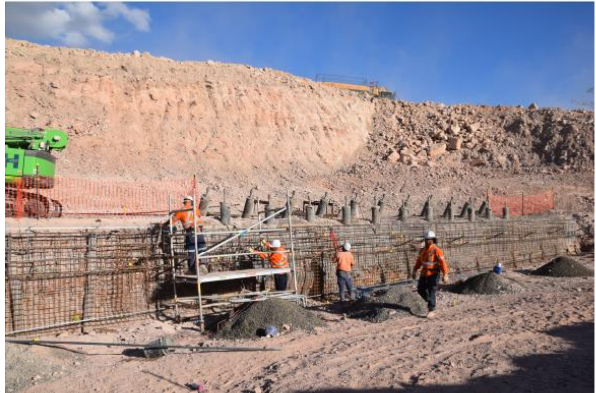
Top section of ROM Slot Wall and Micro Piles
