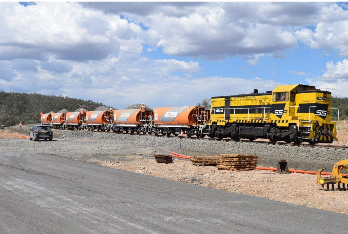
Laying ballast for the rail
