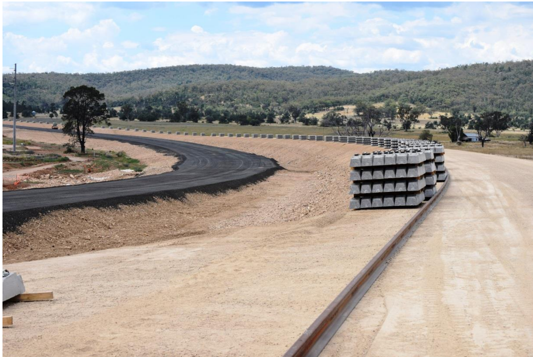
Sleepers and rail line ready for laying
