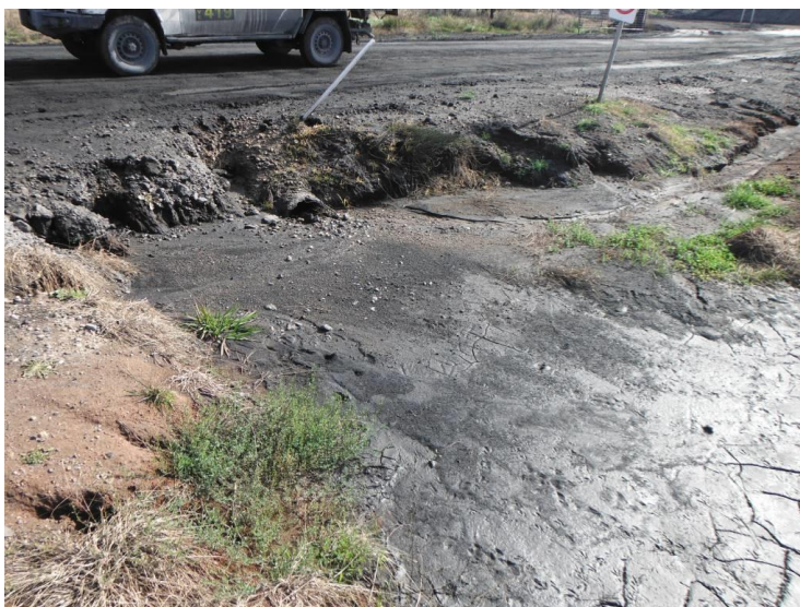
Photo 4 – Built up sediment at culvert. This has since been removed.
