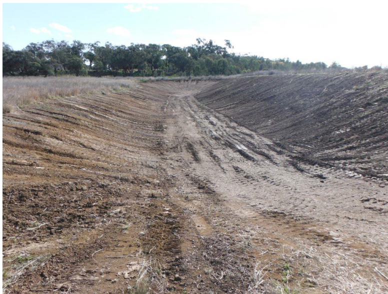
Photo 3 – Reshaped Sediment Dam
