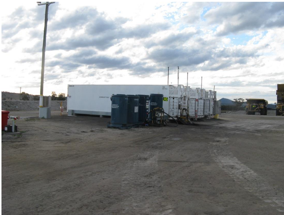
Photo 10: Double lined diesel tanks have been installed at the relocated office and workshop area
