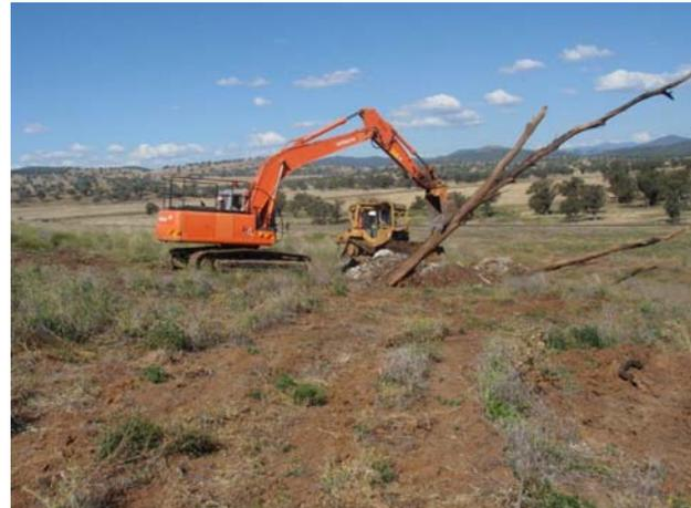
**Plate 7a: Dozer snigging timber on rehabilitation area and 7b: Excavator and dozer installing augmented stag tree in rehabilitation area.**
