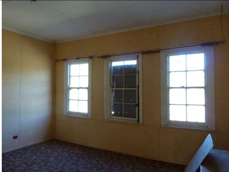
Figure 20 Site H9. Blair Athol Schoolhouse interior. Original schoolhouse windows, wall and ceiling cladding replaced with masonite.
