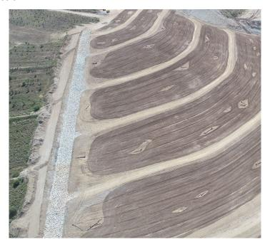
Figure 18 - Photo: Rocklined Drop structure and completed contours on the Southern Rehabilitation area - November 2021.
