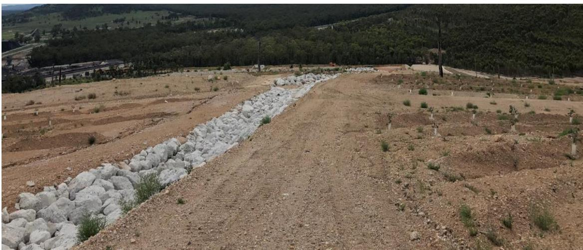
**Figure 17 - Photo: Rocklined Drop structures on the Northern Rehabilitation area**
