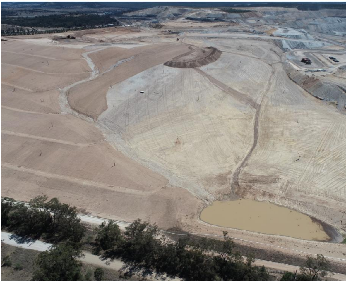
Photo taken in October 2023 displaying topsoil spreading activities on the Southern Emplacement Area
