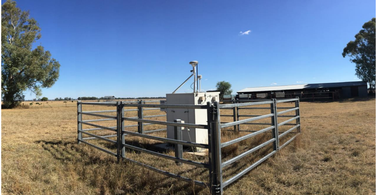
Figure 1: TEOM installed at Flixton property
