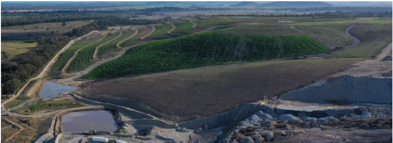
Photo taken in July 2024 showing rehabilitation progression of the South Rehab with fresh vegetation
