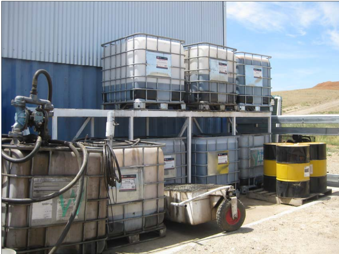
PLATE 5 Oil and Chemical Storage
