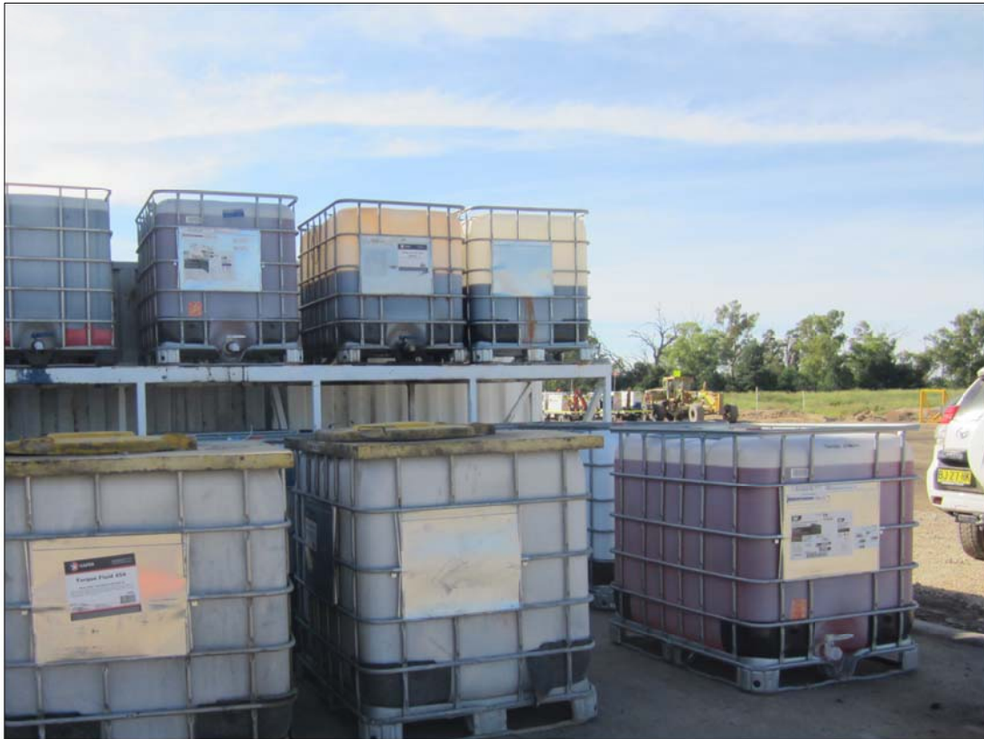
PLATE 3 Oil Storage Compound - note no secondary containment from toppling or leaks under pressure
