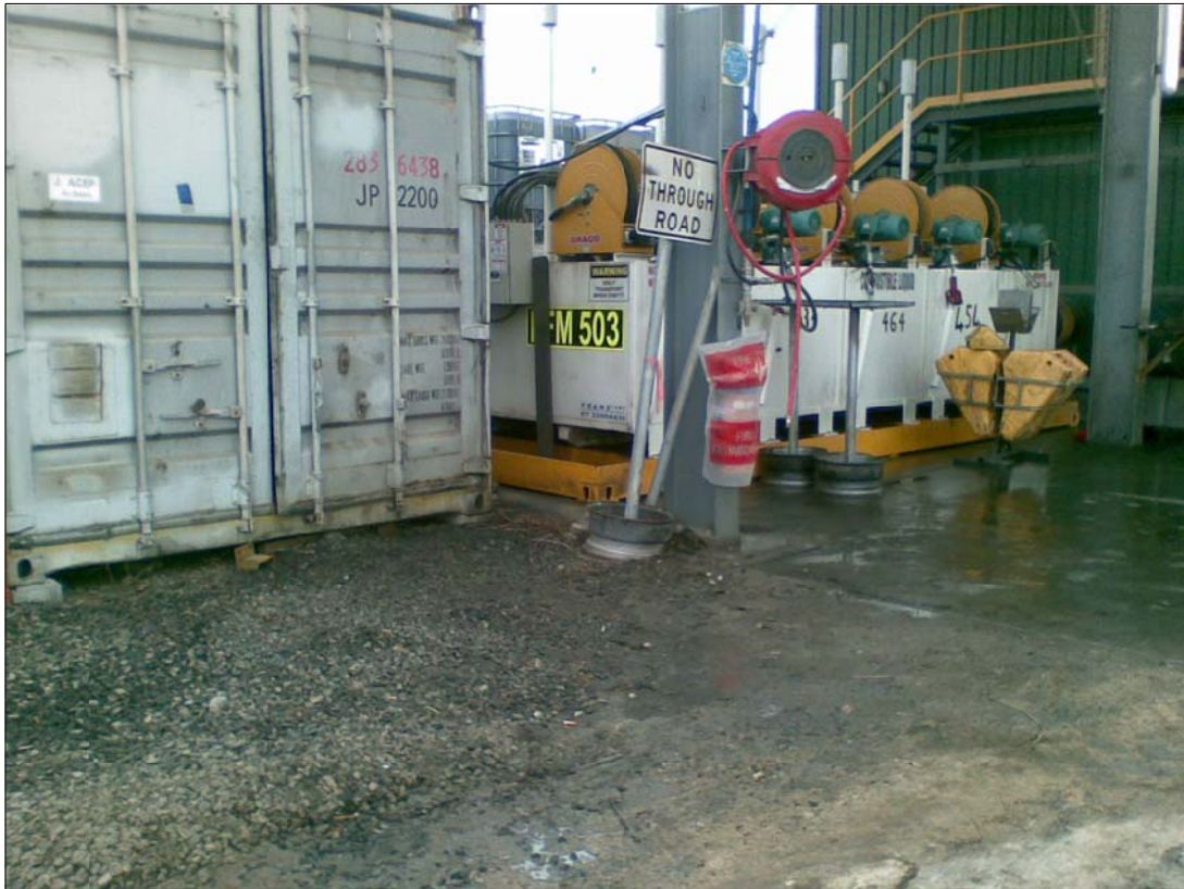
PLATE 1 Hydrocarbon spillage/staining outside waste oil container at workshop
