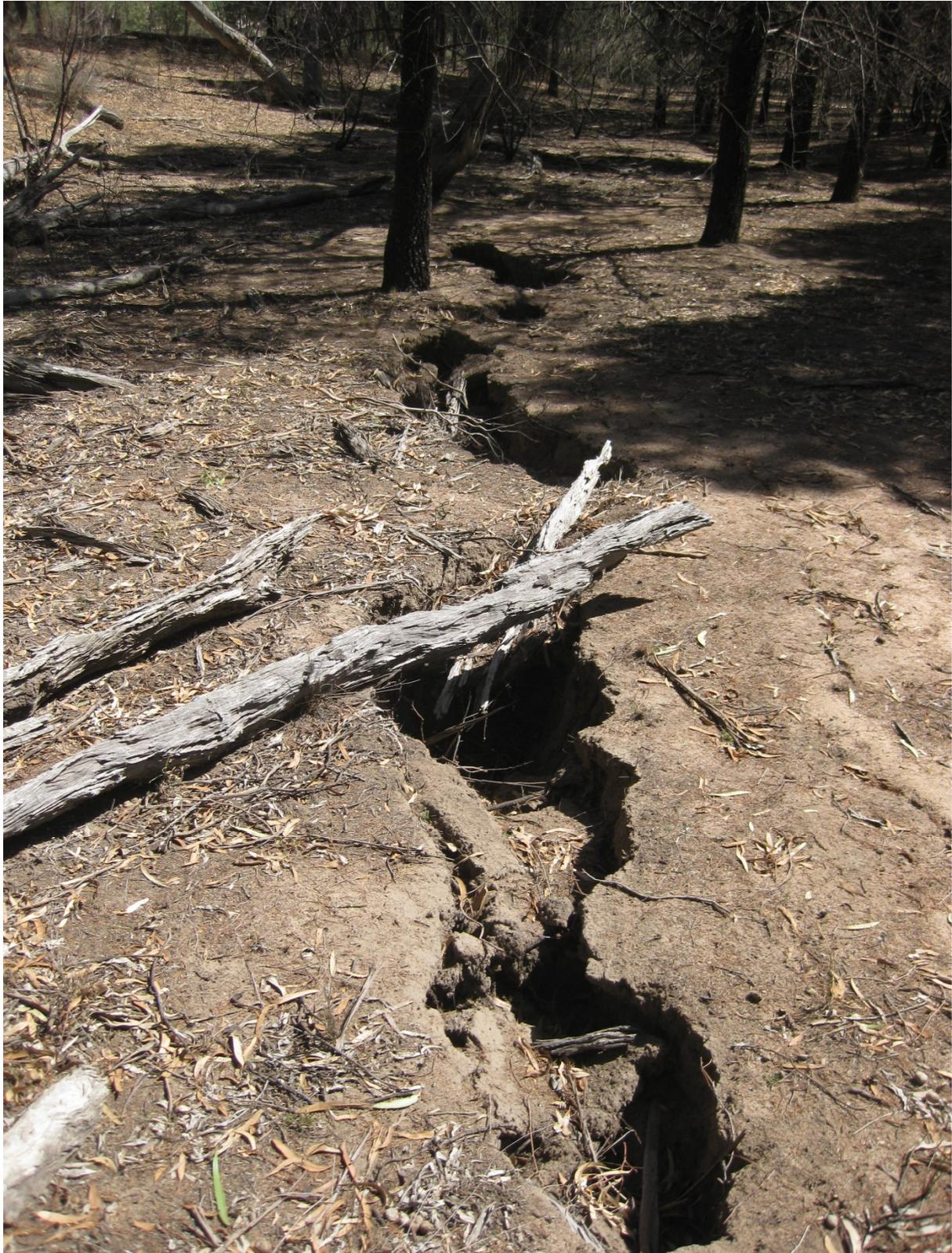
**Photo 12 - Remediated Cracking above LW103 & 104 (ML1609)**
