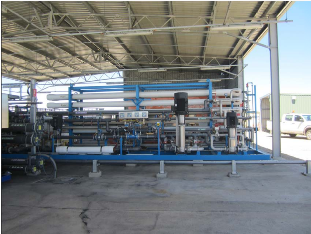
PLATE 7 Reverse osmosis and water conditioning plant
