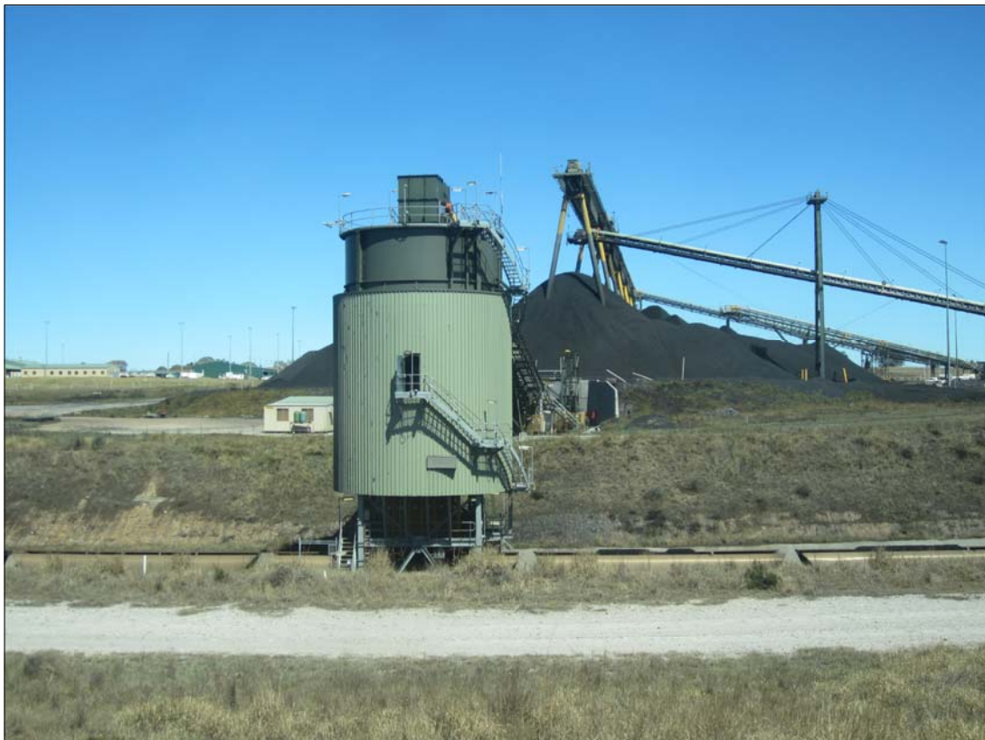
PLATE 5 Product coal stockpile and rail loadout bin
