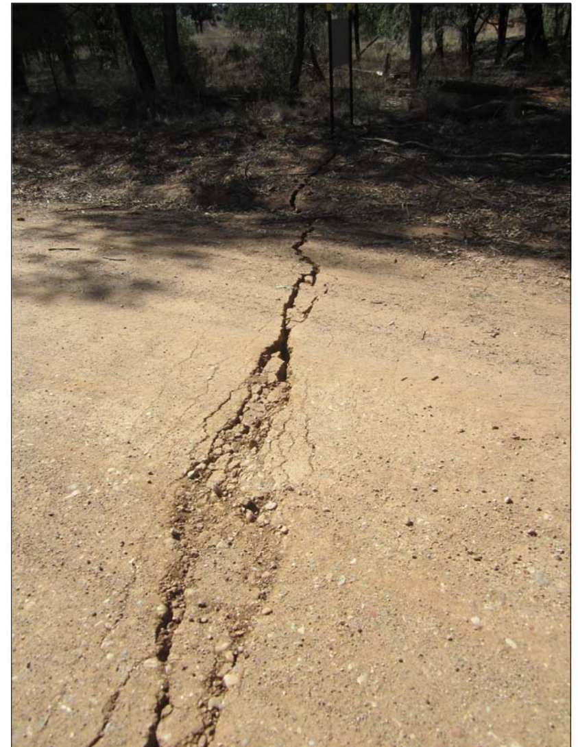
PLATE 10 Cracking across Greylands Road within the subsidence area of LW01 (note: road was closed to public access)
