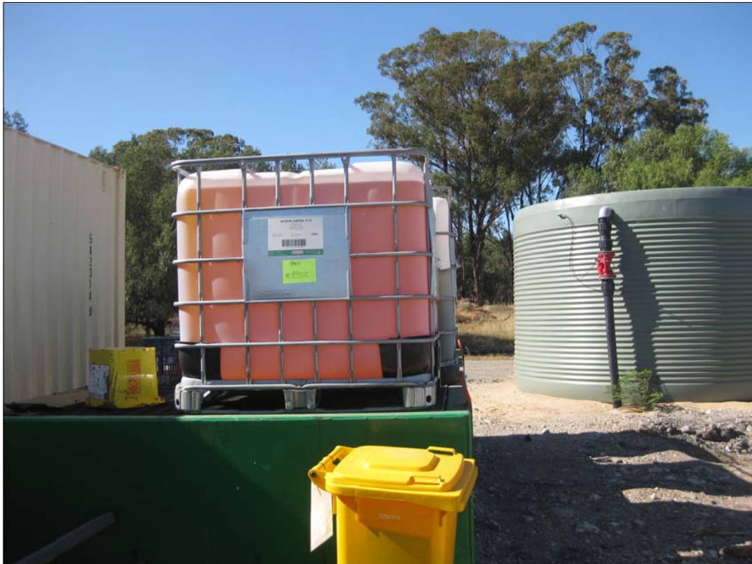
PLATE 1 Storage of Oils and Lubricants at the edge of a Bunded Facility
